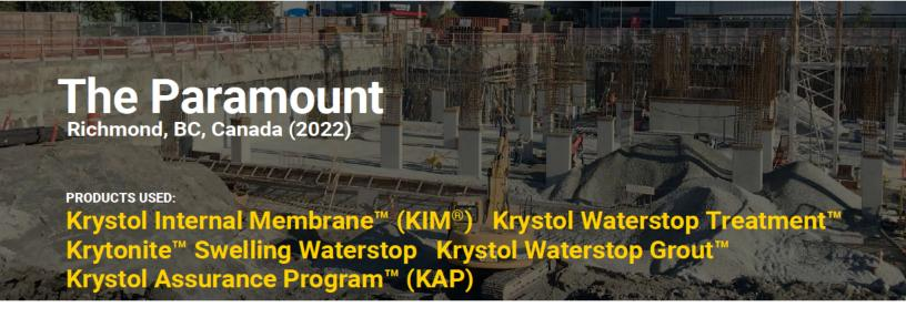
That led the developer to agreeing to a hybrid approach. Instead of applying just one waterproofing product for the highrisk below grade concrete structure, they would use two different systems. One of which would be the traditional externally applied waterproofing membrane system. To negate the impact of that system's vulnerability to tearing, The Paramount construction team would also apply an integral waterproofing system.
