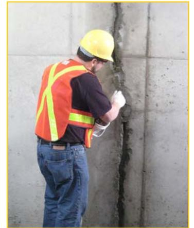
Use the Krystol Leak Repair System to stop water and repair leaking concrete from structures, including:
