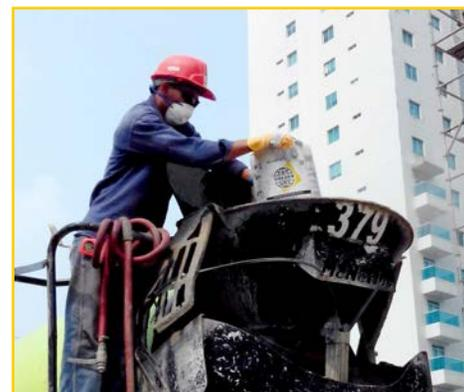
KIM is used to integrally waterproof and increase the durability of concrete subject to water exposure and hydrostatic pressure:
