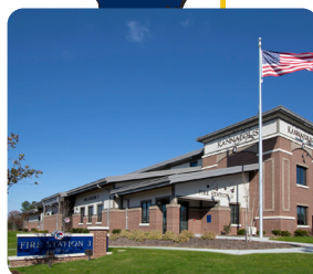
Firestation #3, Kannapolis (Slab) North Carolina
