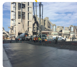
St. Mary's Cement's Alternate Fuels Building>(Slab) Bowmanville, ON
