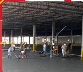
Calgary Bus Barn> (Slab) Calgary, AB
