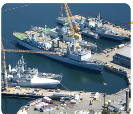
Fleet Maintenance Facility> (Slab) Victoria, BC
