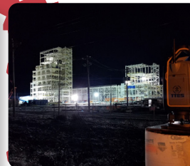
Roquette's Pea Processing Plant (Slab) Portage la Prairie, MB
