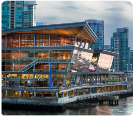
Vancouver Convention Center> (Slab) Vancouver, BC
