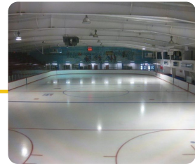
Cole Harbor Place Ice Rink> (Slab) Coal Harbor, NS
