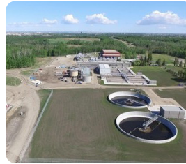
Aquatera's Waste Water Treatment Plant> (Slab) Grande Prairie, AB
