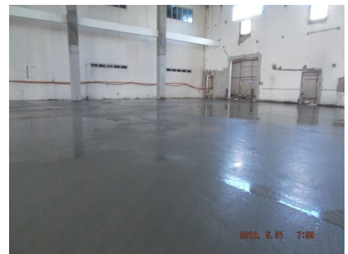
Warehouse Building: 357 m 3 of concrete – 1785 kg of KIM
