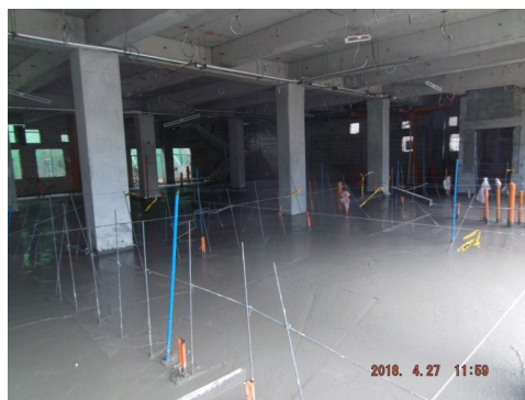
Technical Building: 62 m 3 of concrete – 310 kg of KIM
