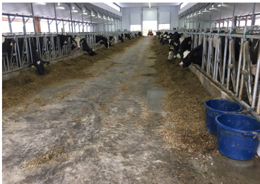
Hard-Cem extends concrete wear life 2-6 times under harsh conditions.
