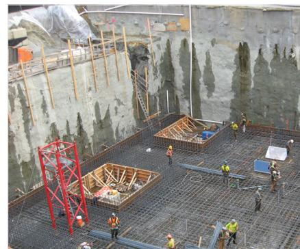
**Laying the rebar for the 1.5 m (1.5 ft.) thick raft slab.**
