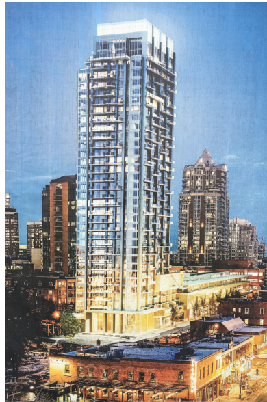
Kryton products waterproofed all the below grade parking areas.
