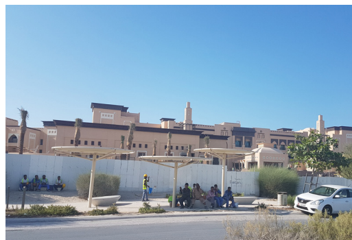
Nearing the completion stage of the Saadiyat Rotana Hotel.
