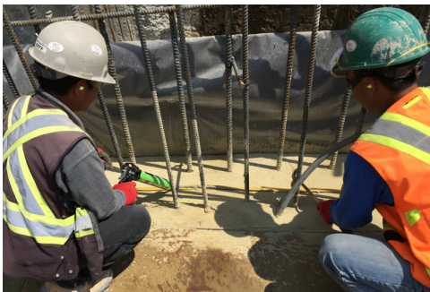
Krystol Waterstop Treatment is applied before the Krytonite Swelling Waterstop. The combination of the two products offers proven long term waterproofing protection.
