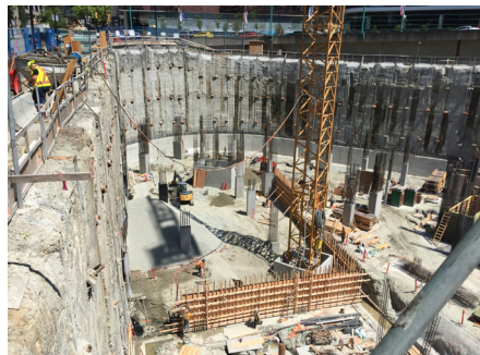
A view into the below grade construction
