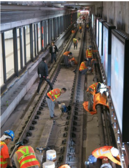
Teams working on waterproofing repairs
