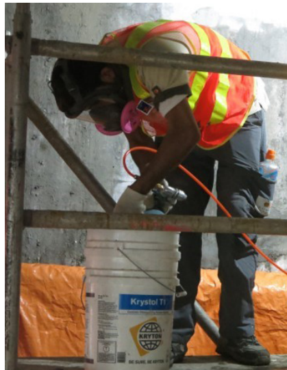
An applicator getting ready to apply T1 to the tunnel wall
