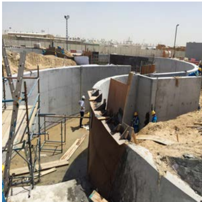
KIM shotcrete and concrete was used to waterproof the canal.
