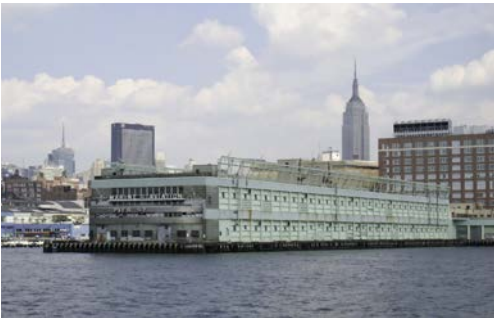
The massive renovation of the Pier required a system that can withstand corrosion and flood waters.
