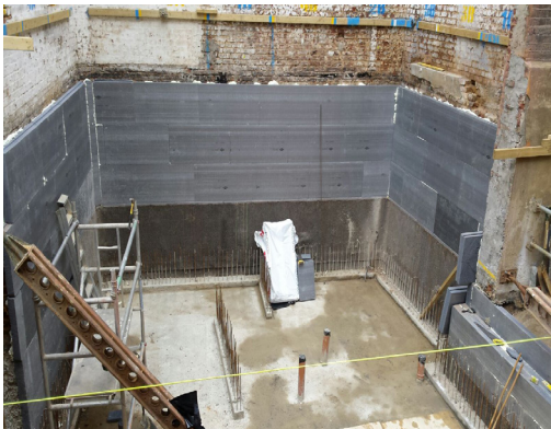
KIM concrete was used for the basement slabs and walls.
