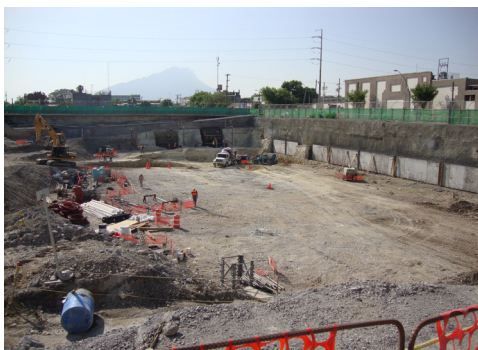
La Capital constructing below grade using KIM to waterproof the shotcrete
