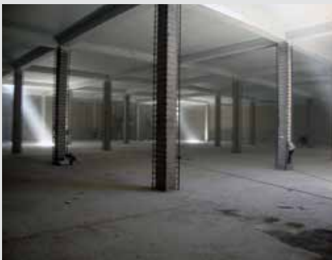
Repair work on the Belenes water tank, Guadalajara, Mexico
