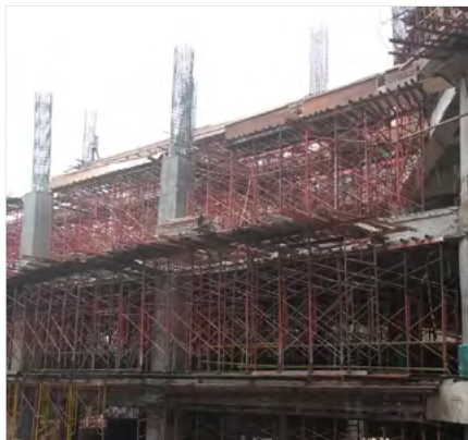
The six story extension under construction.
