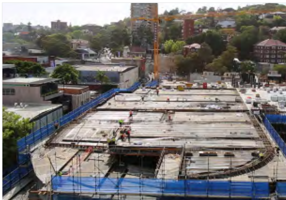
Aerial view of the car park under construction.
