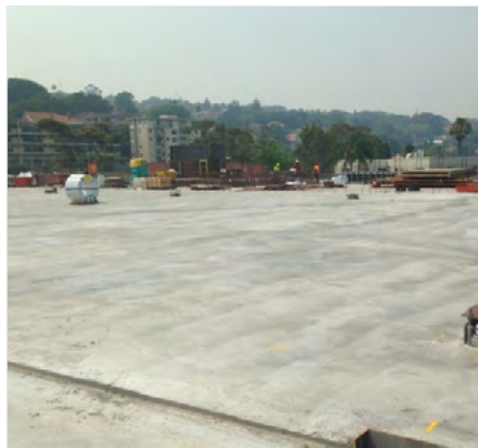
Top level of the waterproofed car park.
