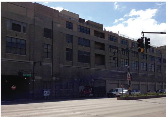
The outside of the Bloomberg building which was hit by major flooding during Hurricane Sandy.
