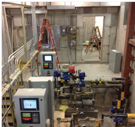
Construction of the new waterproof concrete walls to house important servers for global transactions.
