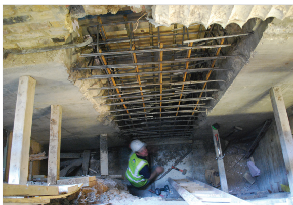
Basement underpinning work.
