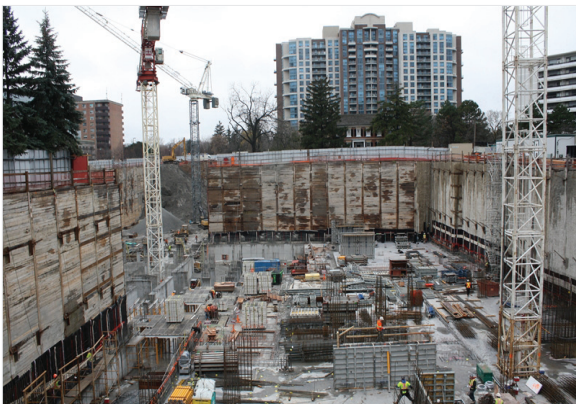
Construction of the three levels of below grade parking.
