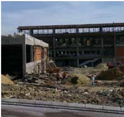
Construction of the mega church.
