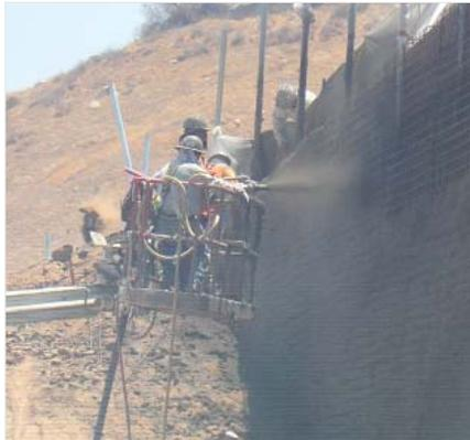
*The applicator for this project, Superior Gunite in Los Angeles, CA, applied Krystol Internal Membrane (KIM) as a method of waterproofing on the wall using shotcrete.*
