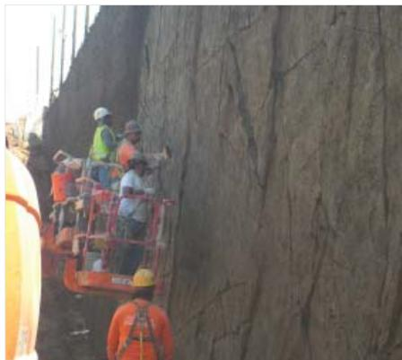
*One shotcrete nozzleman sprayed while four followed closely behind to start sculpting the concrete into the façade.*
