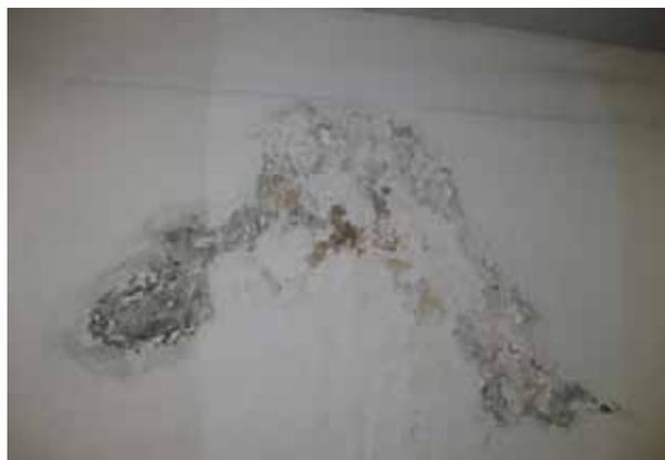
***Mold and moisture was a problem at the site because no waterproofing was done during initial construction.***
