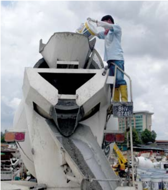
Using KIM makes waterproofing concrete a quick and easy process that does not impede construction timelines.
