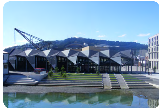
The Te Wharewaka O Poneke Building was developed on reclaimed land along the waterfront in central Wellington, making waterproofing essential.
