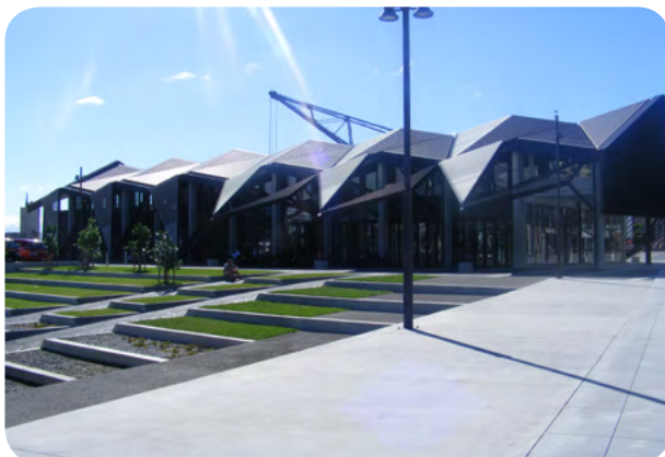
Marine grade concrete steps leading into the lagoon protected by KIM admixture.
