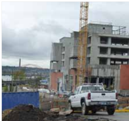
Construction at Brewery District, overlooking the Fraser River.
