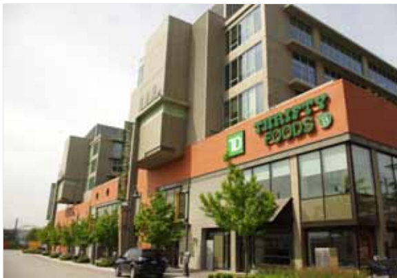
Completed Brewery District project with bridge in the background.
