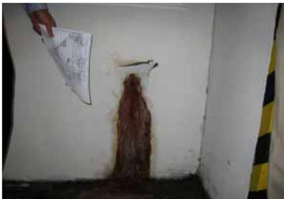
*Just one of the several leaks that The Mall owners were unable to repair using epoxy and other repair systems.*
