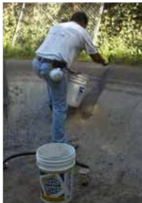
Filling cracks on the tiger pool.
