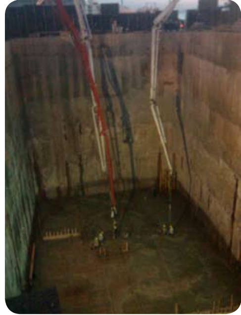
The tall retaining walls made waterproofing a challenge.
