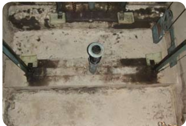
The Krystol Crack Repair System stopped the leaks
