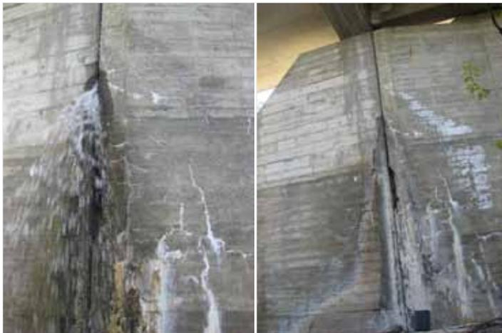
**Aqueduct over Cayoosh Creek – water was pouring out of the crack before the dewatering occurred.**
