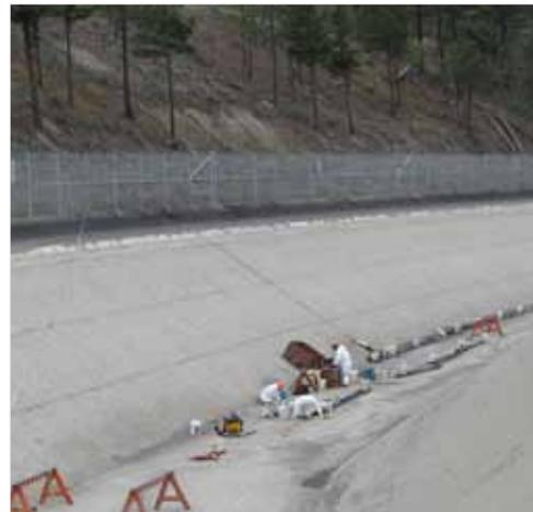
**Workers performing concrete repairs with Kryton products to portions of the canal's walls and floor.**
