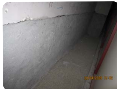
After: The basement walls are all dry, even after heavy rains
