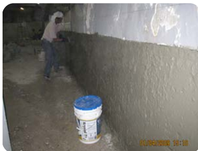
To finish, the repaired wall is coated with Krystol T1
