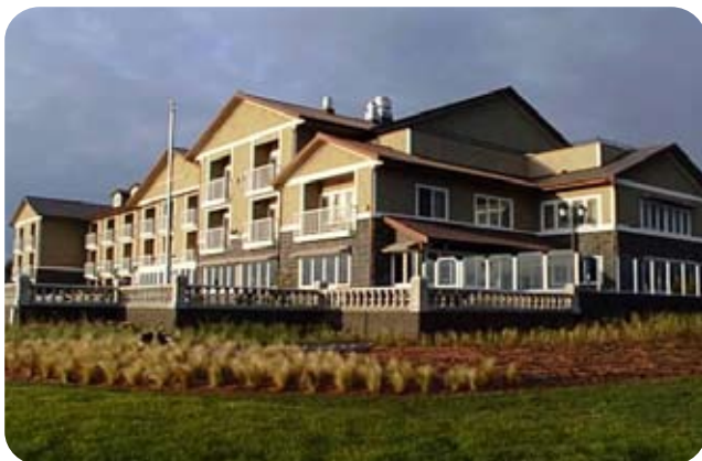
Exterior brick and rock protected with Krystol™ Hydrostop.
