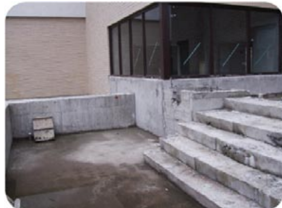
Krystol T1™ and T2™ applied to surfaces of an outdoor pool.
