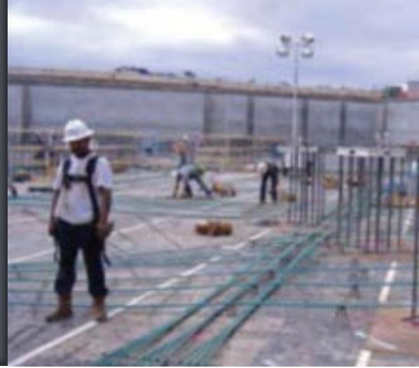
With this distributor, they used about 1,530 m<sup>3</sup> (2,000 y<sup>3</sup>) of shotcrete that incorporated Kryton's KIM, a concrete waterproofing admixture. This allowed them to waterproof all below grade walls and build the water storage tanks for the buildings' sprinkler system. To protect all the construction joints involved in this work, the team also used Kryton's leading jointing process, the Krytol Waterstop System.
