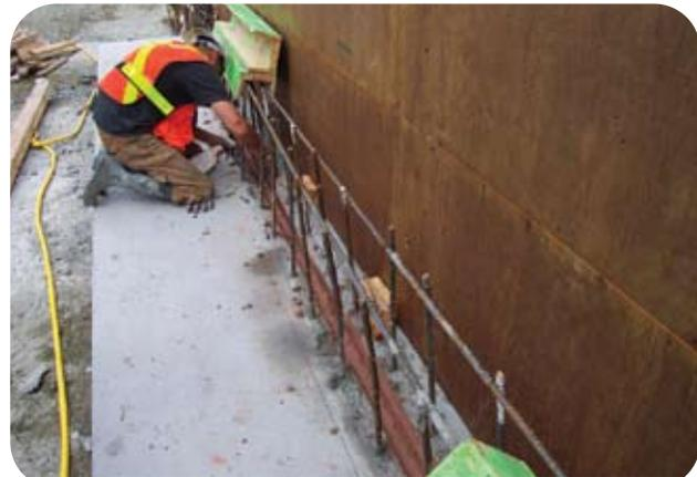
**Above: Krystol Waterstop application to all the construction joints.**
