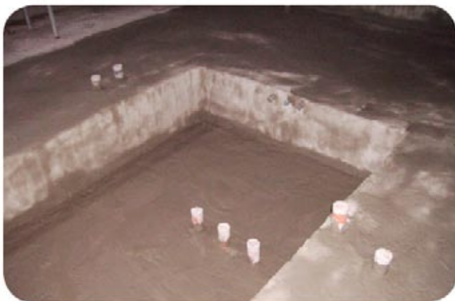
Krytol T1™/T2™ freshly applied to bathroom surfaces.
