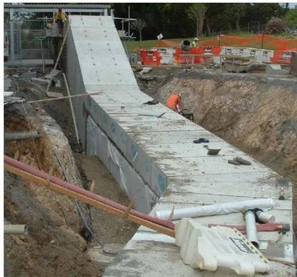
*All fifty of the precast box culvert segments were waterproofed with KIM.*
