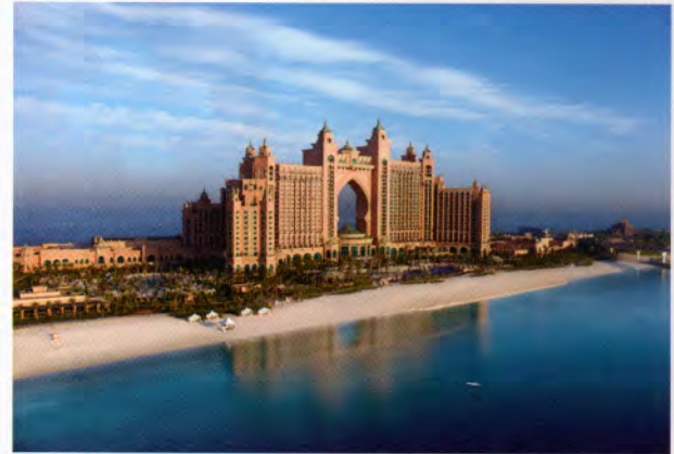
Kryton products waterproofed below grade water storage tanks at the Atlantis Hotel, Dubai
