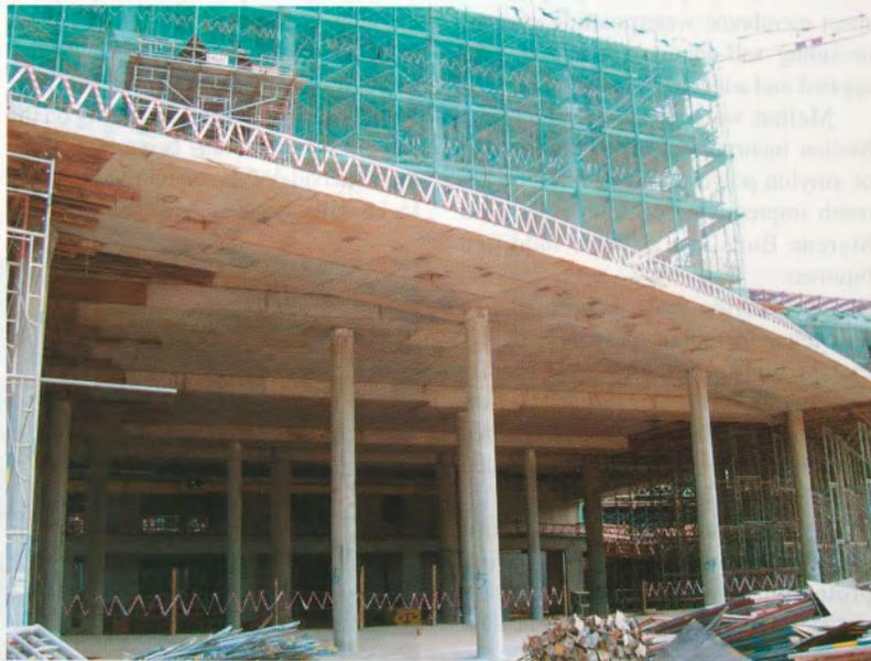
Kryton's Integral Crystalline Waterproofing technology was applied on the Agora, one of the large elliptical concrete decks of the common facilities.
