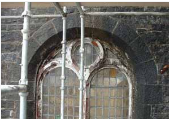
KMA was added to the render to seal all the windows.
