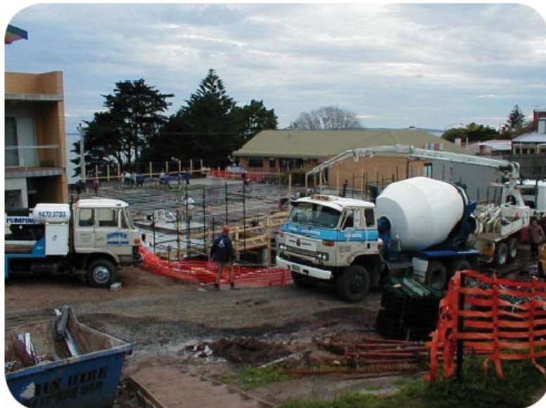
KIM® being mixed on-site prior to pouring
