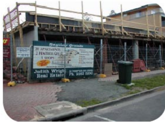
KIM® applied to balconies and slabs.
