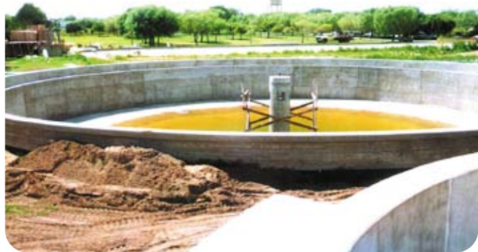
Concrete required excellent chemical resistance.
