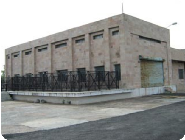
The Sewage Pumping Station, first constructed and subsequently repaired using the Krystol® crack repair system remains dusty dry almost 8 years later.
