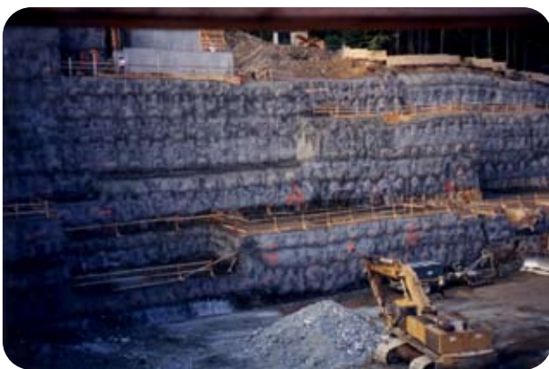
Spring run-off presented a significant waterproofing challenge.
