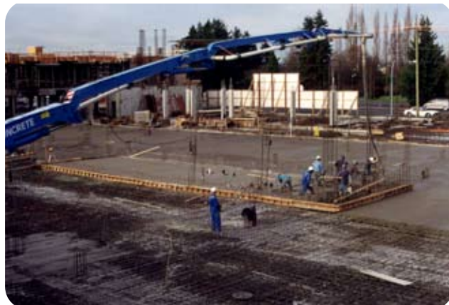
KIM™ used in enormous slabs below sea level.
