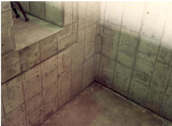
*The Fraser River's water pressure caused leaks in the Pipe Plant.*
