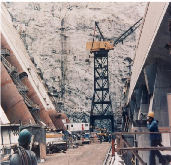
*Kryton Krystol T1® & T2® Waterproofing system was used to waterproof the exterior face of the powerhouse wall.*
