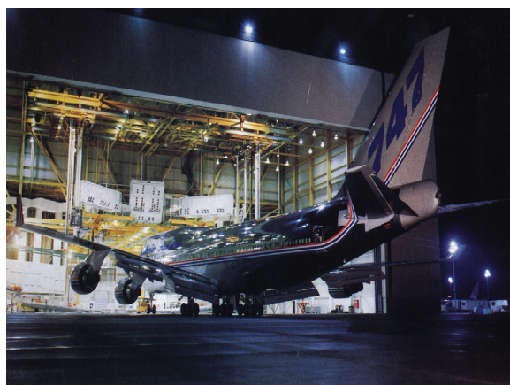
The Boeing Development Center is the largest building by volume in the world.
